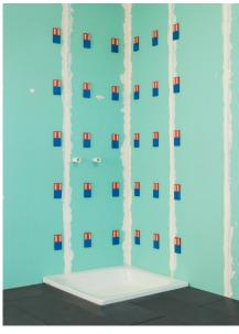
Installing a rear shower wall by means of the key and lock principle
