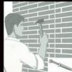
Fix the panels using screws with incorporated plugs. Each panel needs around 15 to 20 screws.
