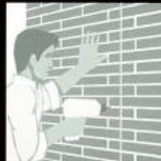
Put the panel on the surface and drill (only in joints between bricks, never in bricks) with a 6mm bit.
