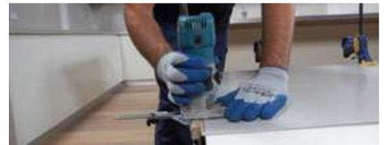
3. The slight overlap of the fold is retained to allow for the thickness of the double sided tape and silicone fastening to the wall.
